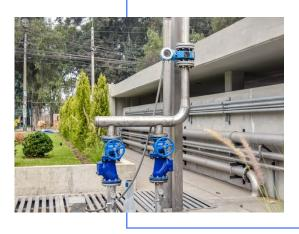
As part of the new WWTP project, we have implemented an innovation where  $CO_2$  emissions from the boilers are channeled to the neutralization tank. This process allows the  $CO_2$  to react with the effluent, forming carbonic acid, which lowers its pH. This technique reduces the amount of chemicals needed for pH neutralization and, in turn, reduces GHG emissions.
